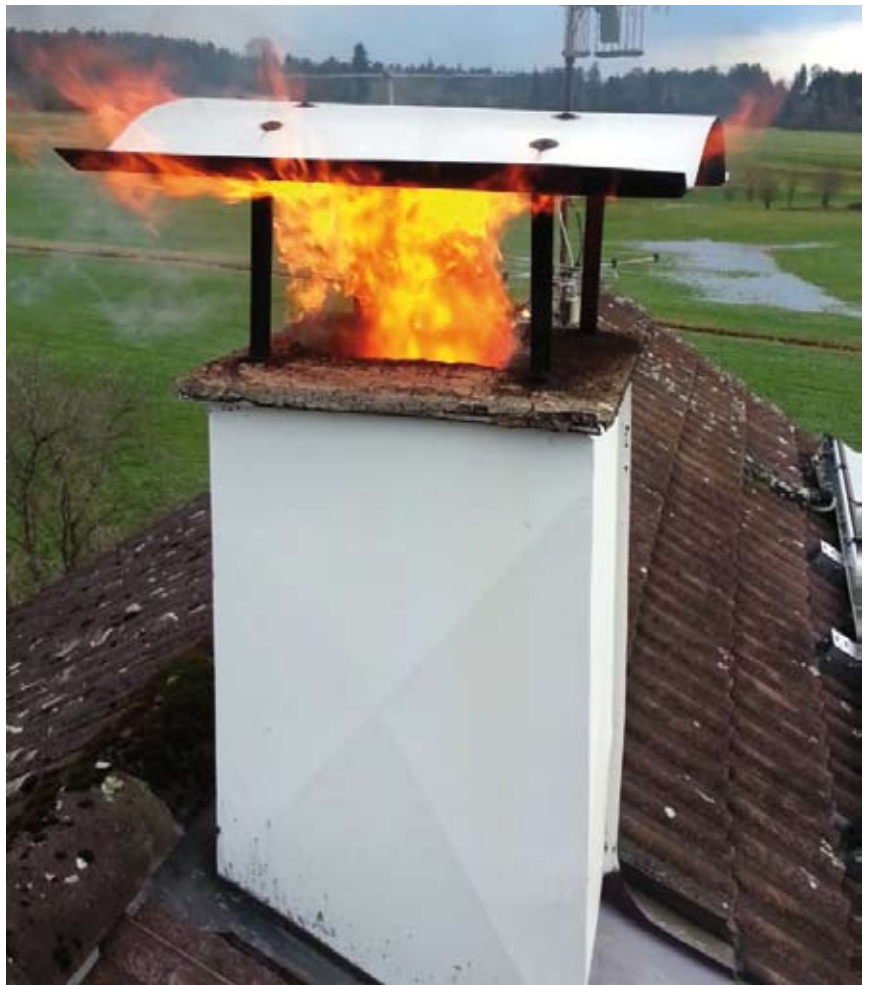
Combustible residues in exhaust or ventilation systems can lead to damage fires
