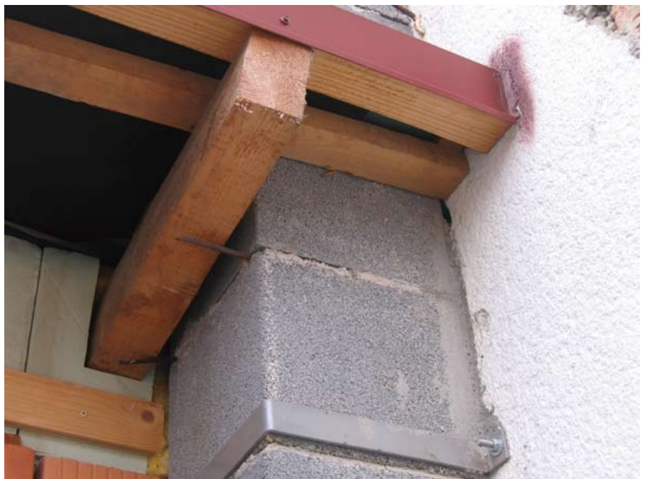
Too small distances to combustible components (Picture ARGE ESCHFOE)
