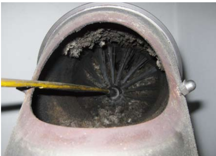
Cleaning a connecting flue pipe via the cleaning opening in the pipe bend
